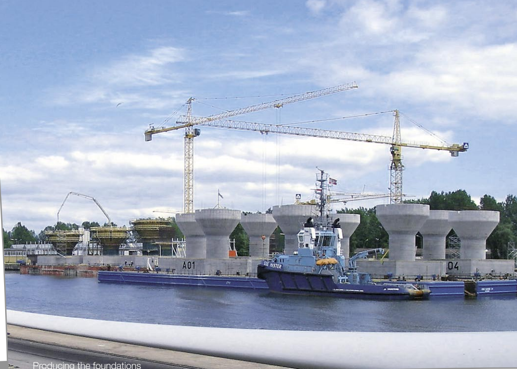
Producing the foundations
