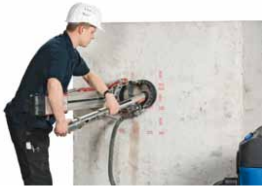
Inserting the undercutting head into the core hole.
