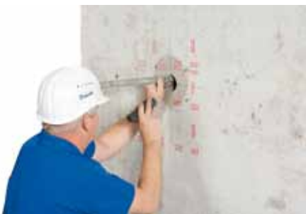
Checking the completed undercut with a special gauge.
